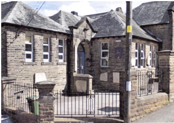
Secondary Modern School at Nabb now Holmfirth J.M.I. and Nursery School
