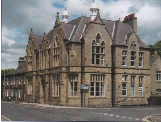
Holmfirth Secondary Modern School and Technical Institute, at time of writing Further Education Centre
