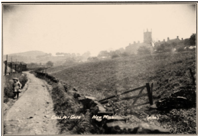
Coal Pit Gate, New Mill 1910 1
