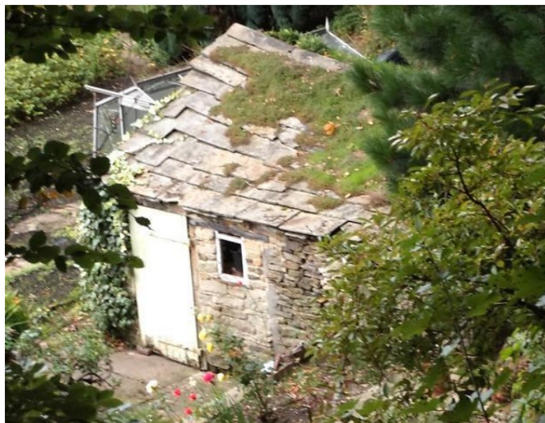
The building used as the pony shed at Sinking Wood Pit, New Mill
