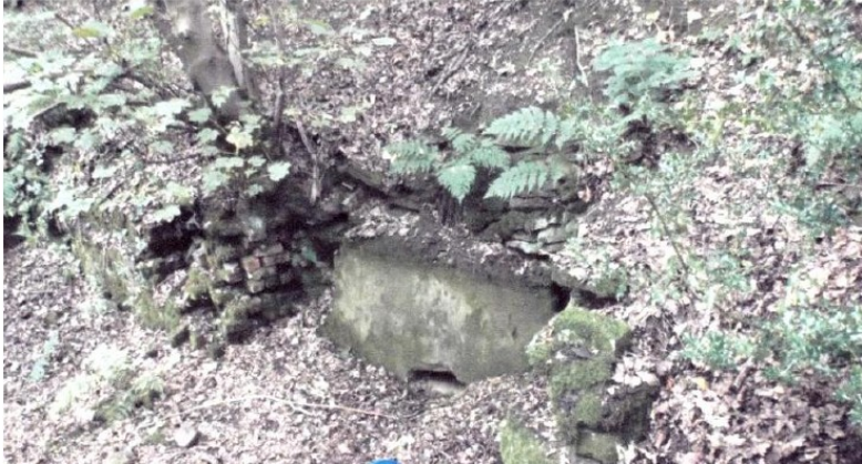
The sealed entrance to a drift mine in Sally Wood, New Mill 2013
